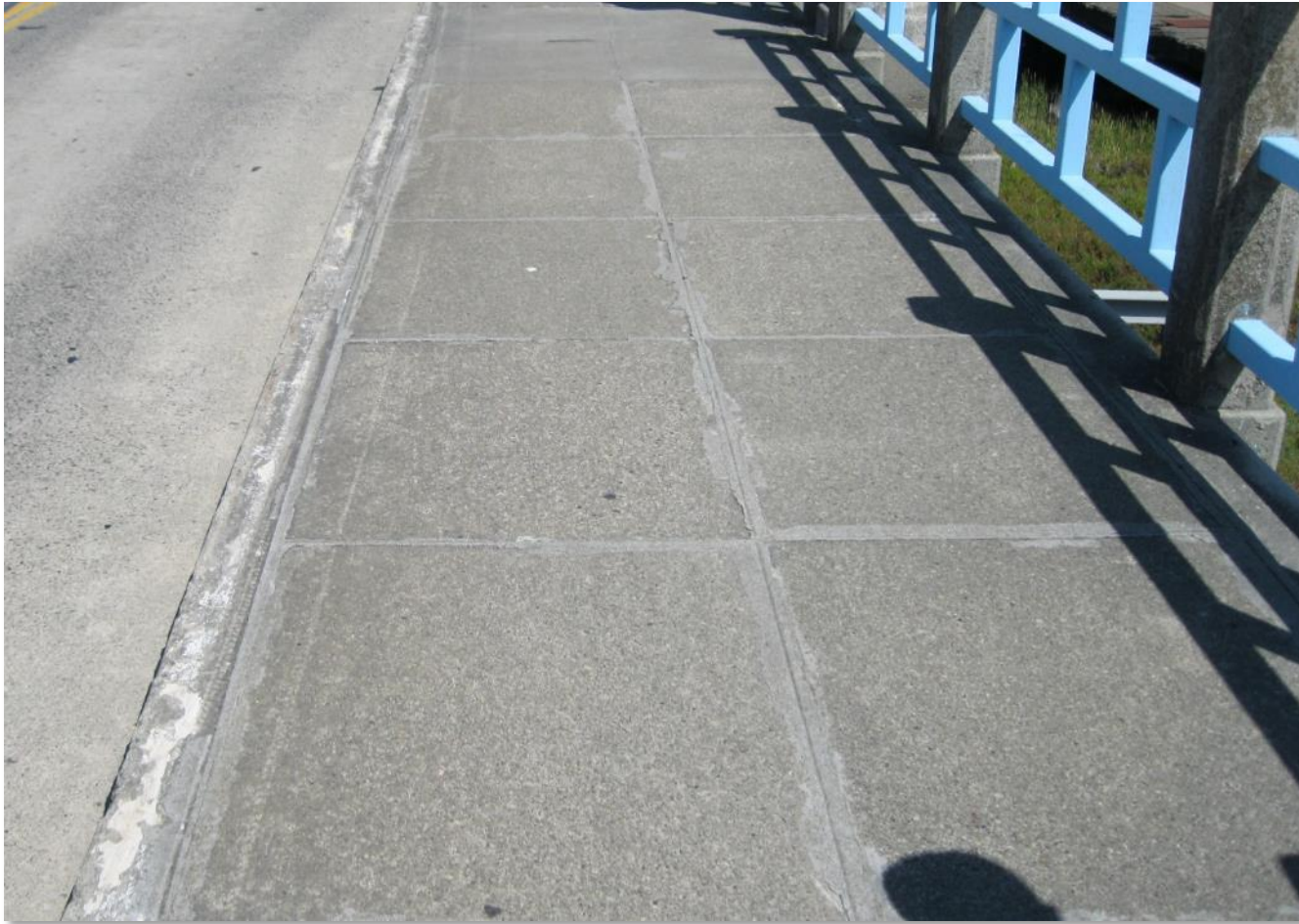
Sidewalk replacement with Precast Panels
