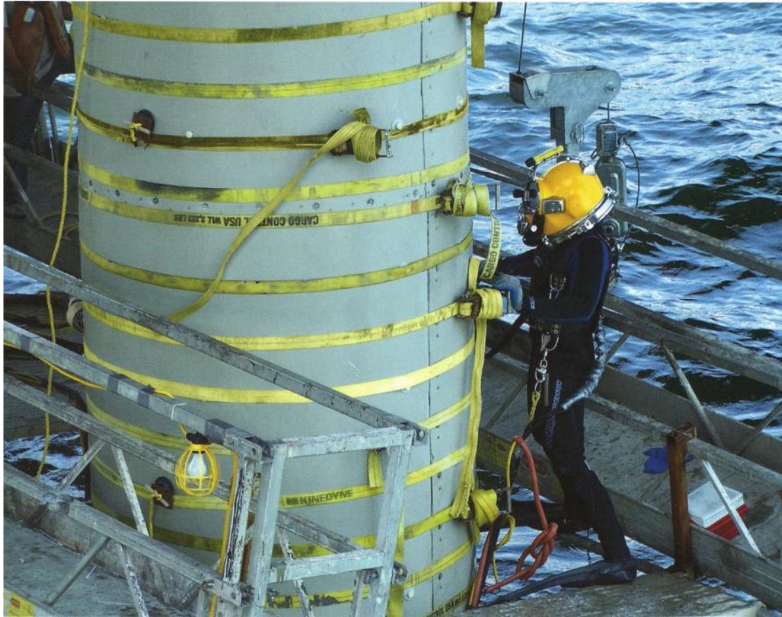
Concrete and Rebar Repair & Jacketing
