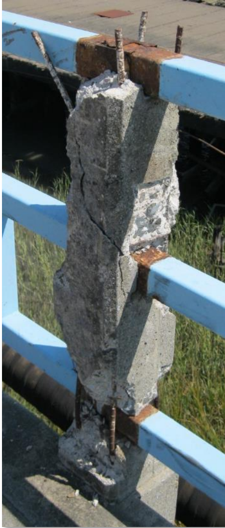
Complete Post Replacement
